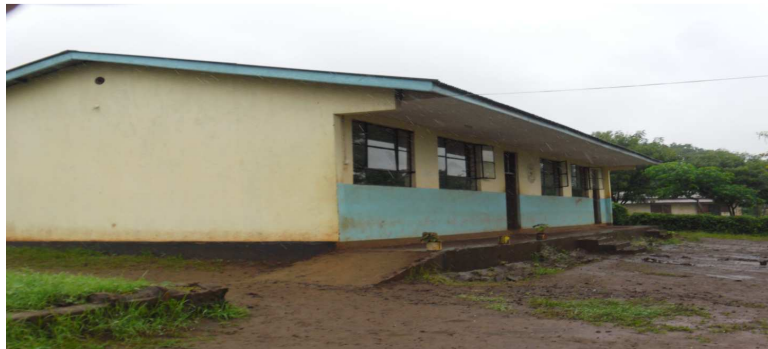
PLATE 2: TWO TASAF CONSTRUCTED CLASSROOMS AT MANGI MAREALE SECONDARY SCHOOL
