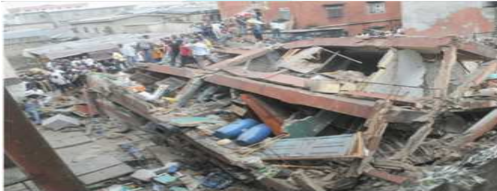
FIGURE 2.2 IMAGE OF A SIX STOREY BUILDING THAT COLLAPSED IN LAGOS, NIGERIA.
