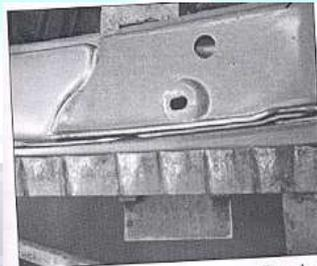
**FIG.7 INSERTION OF 2MM SHIM AND IMPROVED CLAMPING**
