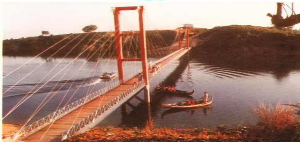
Hanging Bridge at Rangamati
